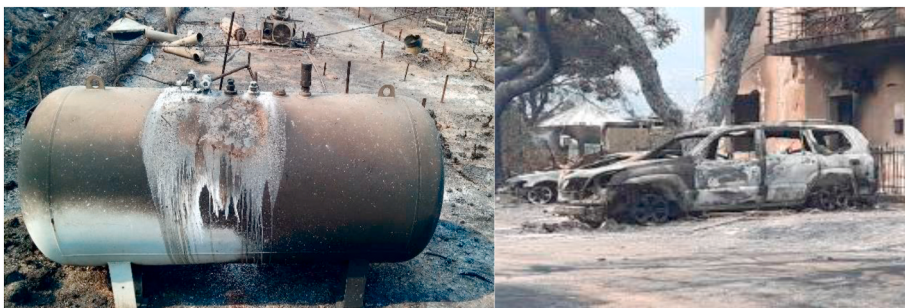
Fig. 6. Burned tanks with Liquified Petroleum Gas (LPG), also cars and trucks and the melting of the aluminum parts, wheel rims and car windows is indicative of the high temperatures developed during the course of the fire [26].
